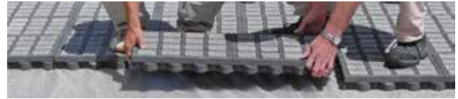
Laying of the filled TTE® elements in twos
