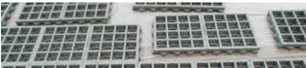
Laying of the TTE ® elements on the fine matrix (installation aid)
